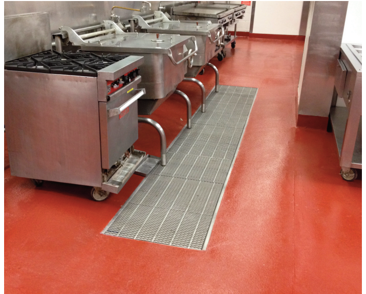
A seamless polyurethane system using Stonclad UT and Stonset TG6 provides The El Paso County Jail with protection from moisture, impact, abrasion, chemical spills, and thermal shock. It’s an ideal floor for a commercial kitchen’s harsh environment.
