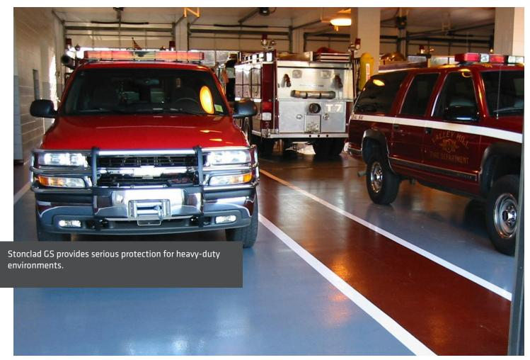
This seamless, epoxy resin system with polished aggregate is impact, abrasion and chemical resistant. A seamless cove base provided a smooth transition between the floor and wall.
