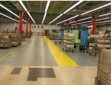
system cures to an extremely hard mortar which exhibits excellent wear properties.
