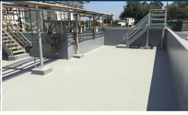
High-performing resin chemistries provide exceptional lining protection for ultra-corrosive environments and perform under extreme physical conditions. The Stonchem product line leads the industry in protection for secondary containment, processing areas, chemical storage, and battery rooms.
