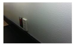
**ROLLER MARKS / EXCESSIVE TEXTURE** • Low ambient temps during application.
